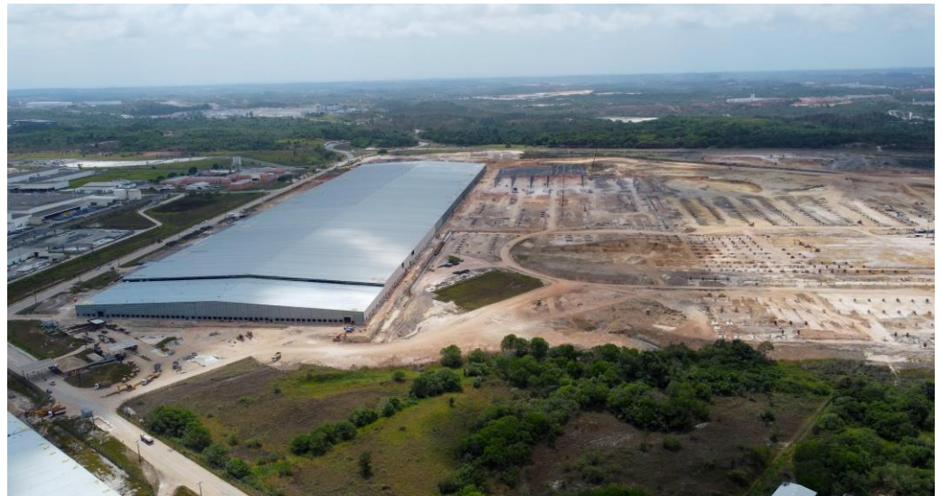
Construction work on the BYD Brazil factory in Camaçari (BA)
